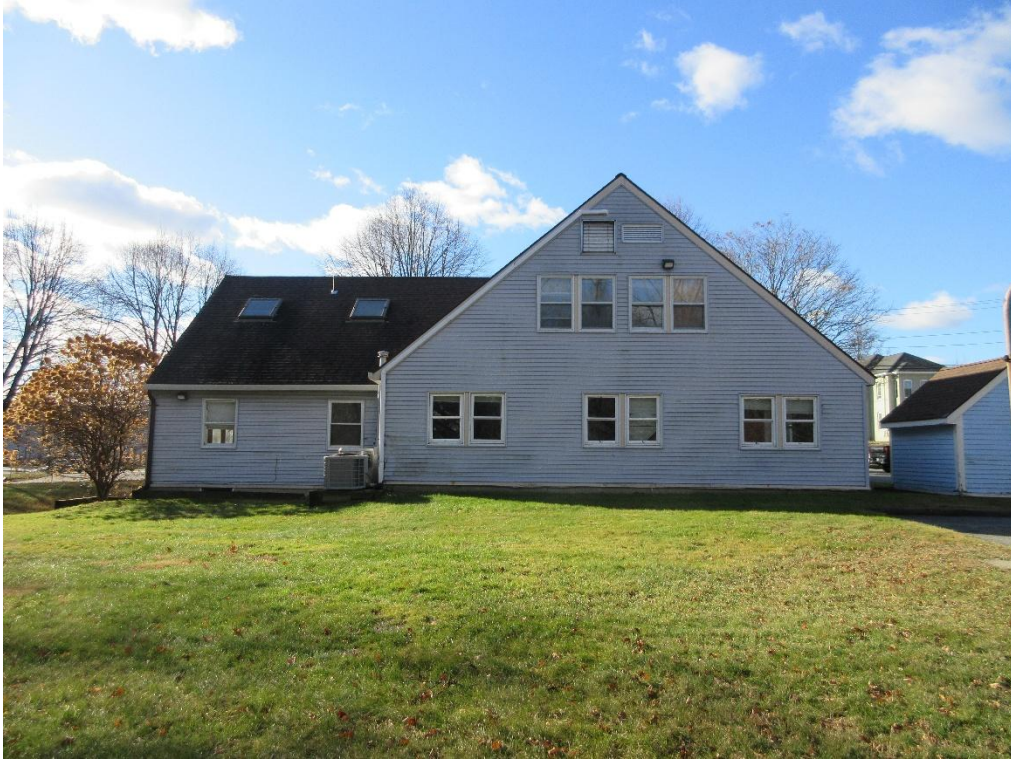
East Side of the Building
