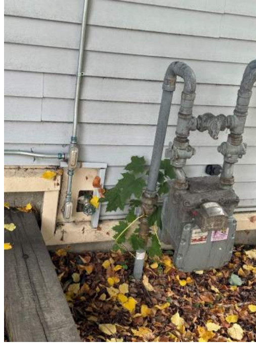
Figure 25-Natural Gas Meter
