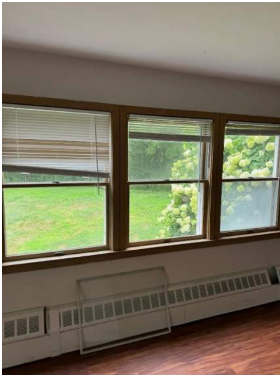
Figure 4-Typical Baseboard Radiation
