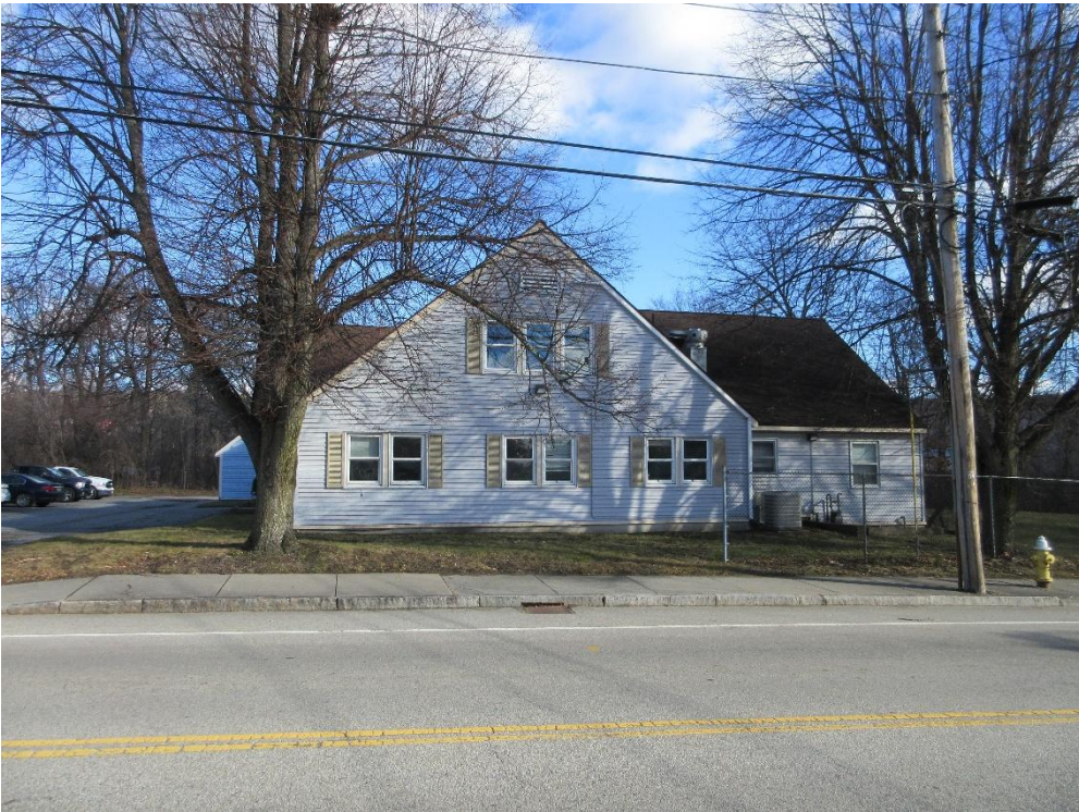
West Side of the Building
