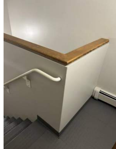
Stair A Second Floor Landing
