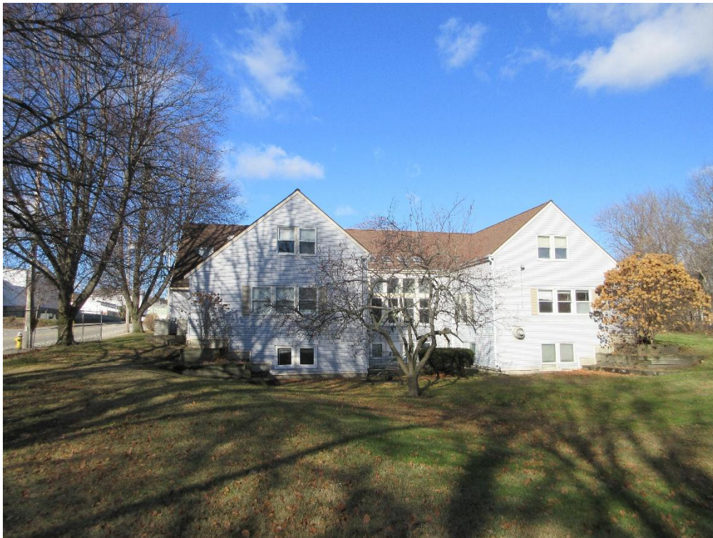
Rear (South Side) of the Building
