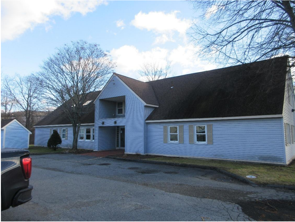
Front (North Side) of the Building
