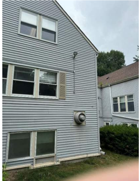
Figure 7-Grease Exhaust Fan
