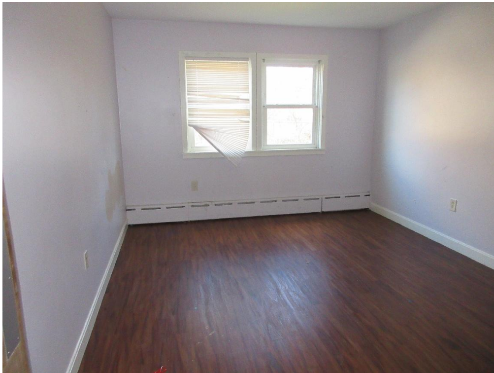
Sample Interior of the Building
