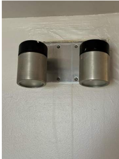
Figure 20-Older Emergency Light
