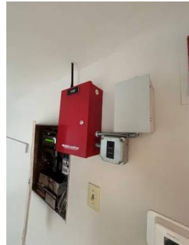
Fire Alarm Control Box
