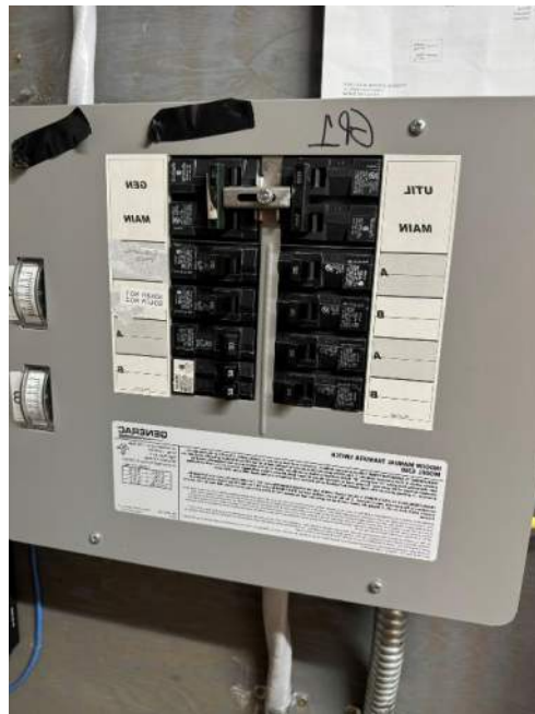
Figure 15-Manual Transfer Switch
