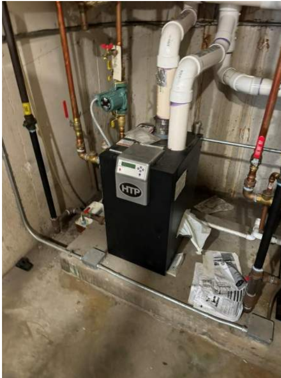
Figure 2-Condensing Boiler 1
