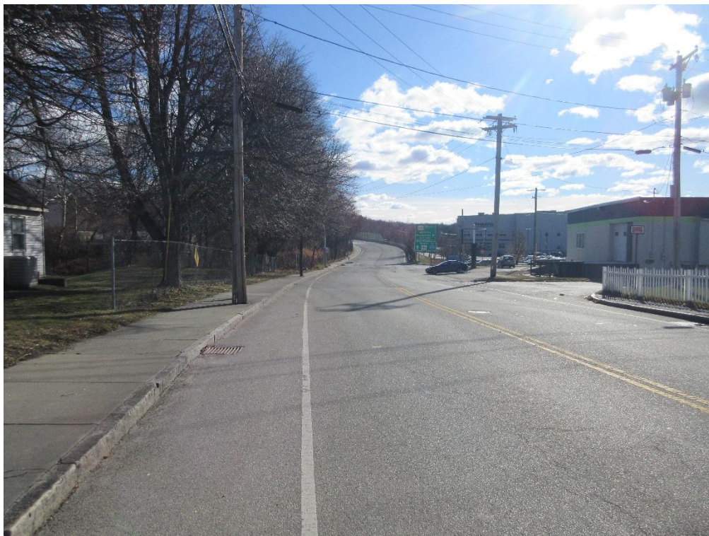
Facing Southeast on Blackstone River Road
